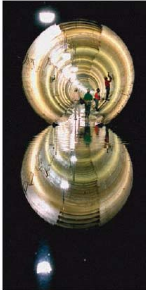
Terminated Texas tunnel The SSC was abandoned after about 25% of the tunnel for the 87-kilometer-circumference large collider ring had been bored.
