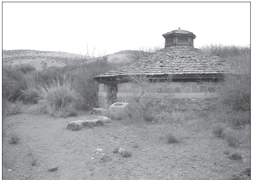
Cooke’s Spring. This spring was heavily utilized during trail days. The spring was later covered with this structure by the railroad. Fort Cummings is located nearby. Photo by Cam Wade.
